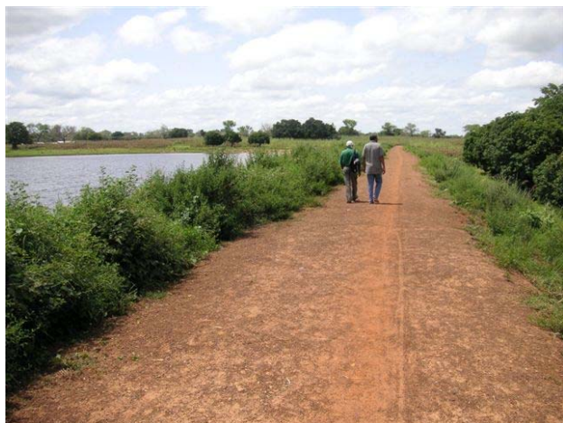
Picture 2: Small Reservoir and dam Upper East Region in Ghana (Source: Schuetz, 2005)
